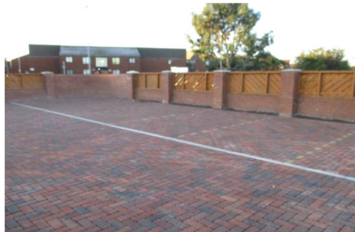
After: New Parking Area to rear of Alice House
