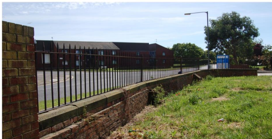
Before: Waste Ground Area to rear of Alice House
